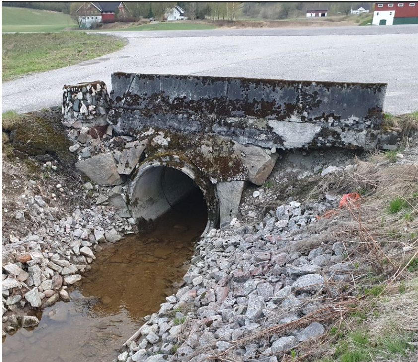
Figur 17: Kulvert under Rv. 36
